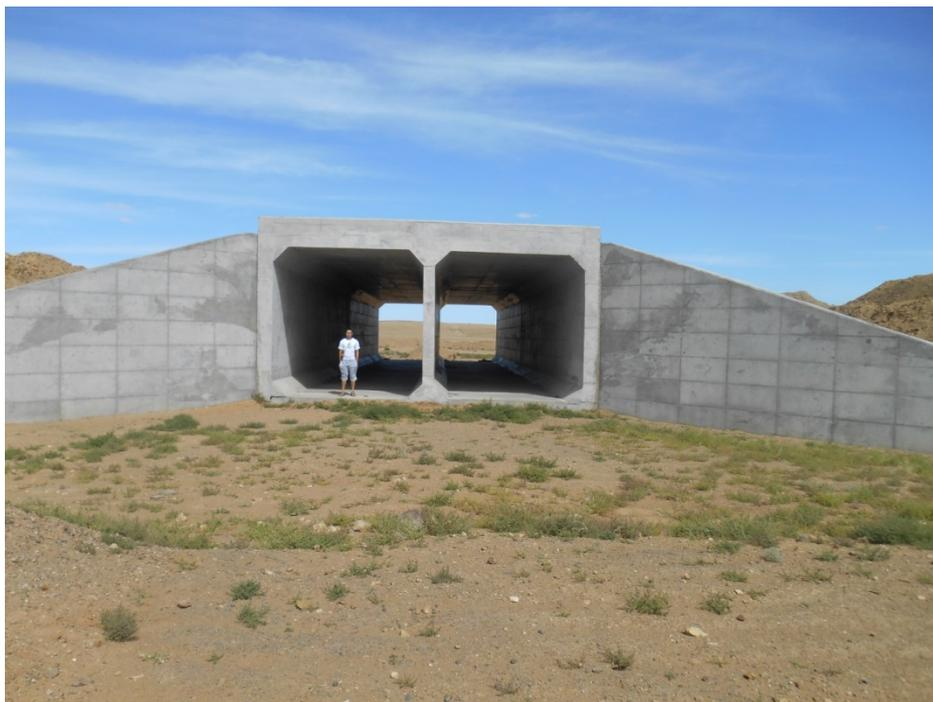
**Figure 22: Double Box Culvert along Partially Constructed Railroad**
