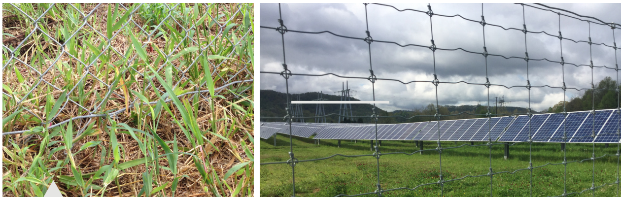
Comparison of a standard chain-link fence (left) with a wildlife-permeable fence (right). © Liz Kalies/TNC
