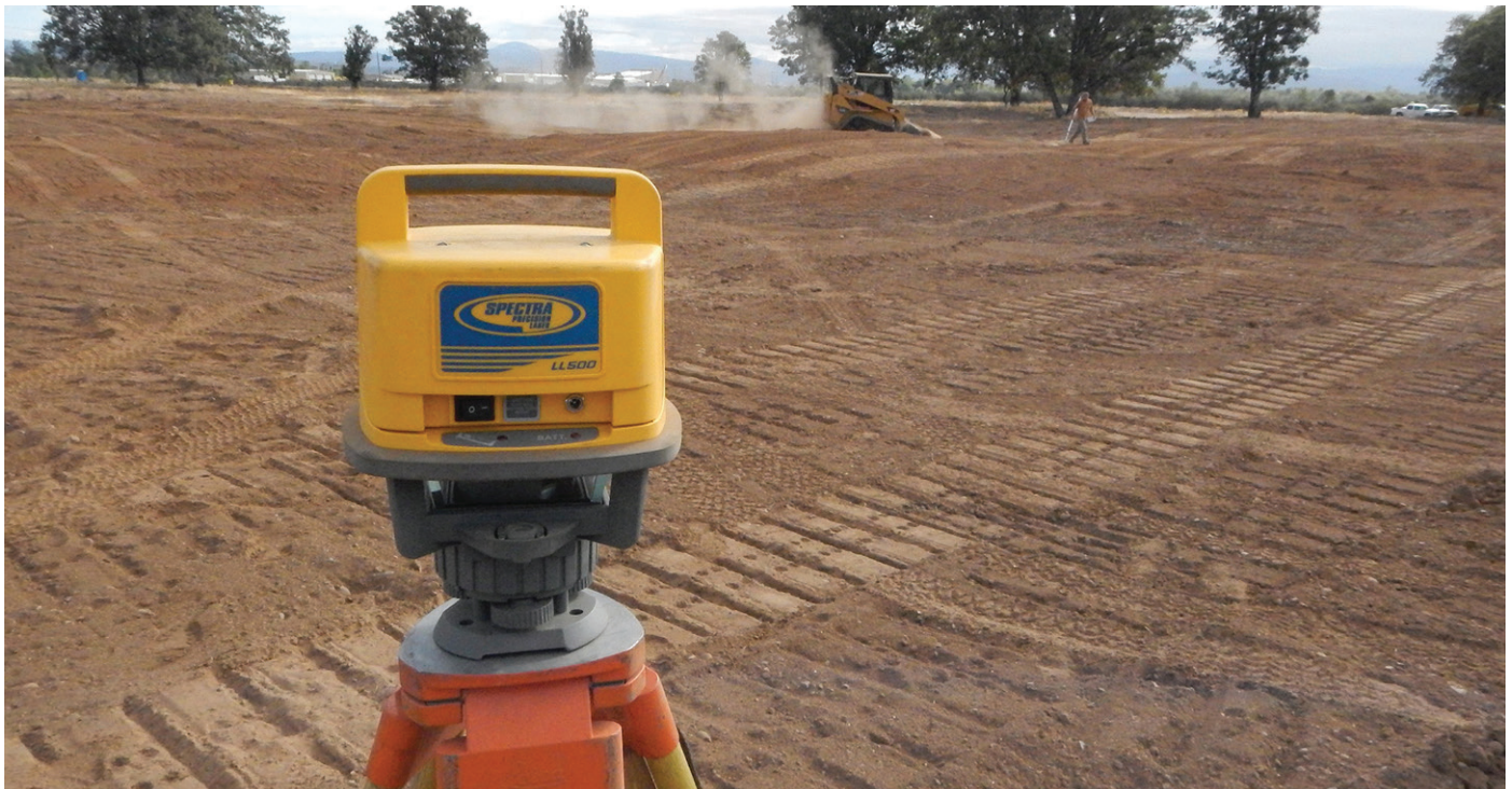
Surveyor's laser level in use for precise relative elevation measurements across a series of newly excavated vernal pool basins during grading checks. Background: a track loader builds up an outflow invert to increase basin depth. © Karen Hussey/TNC
