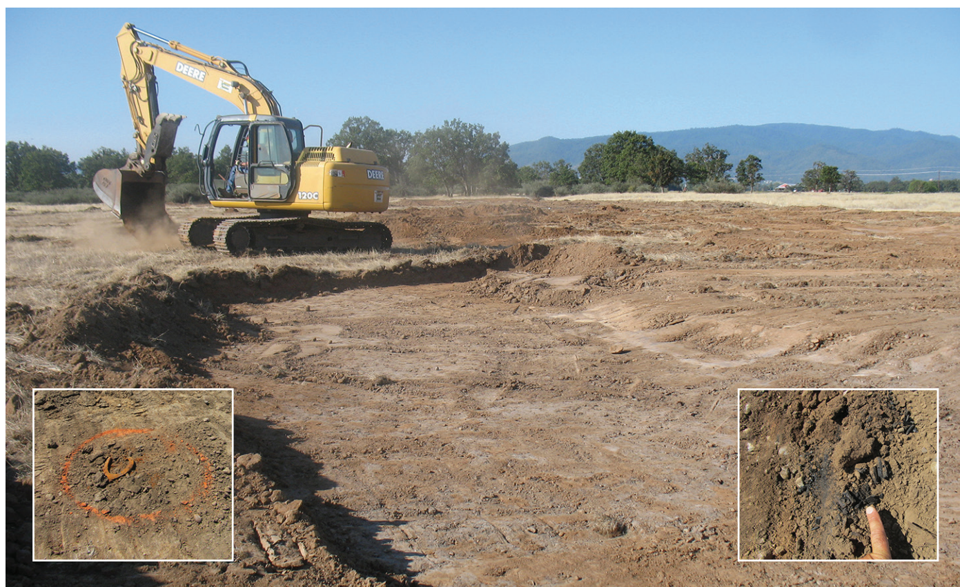
A buried surface of gray wetland Winlo soil is revealed as excavation removes several inches of rust-red upland Agate soil fill from a vernal pool basin during restoration grading. Insets: horseshoe artifact (left) and buried charcoal (right) uncovered at the wetland soil surface provide further evidence of the historic terrain.
