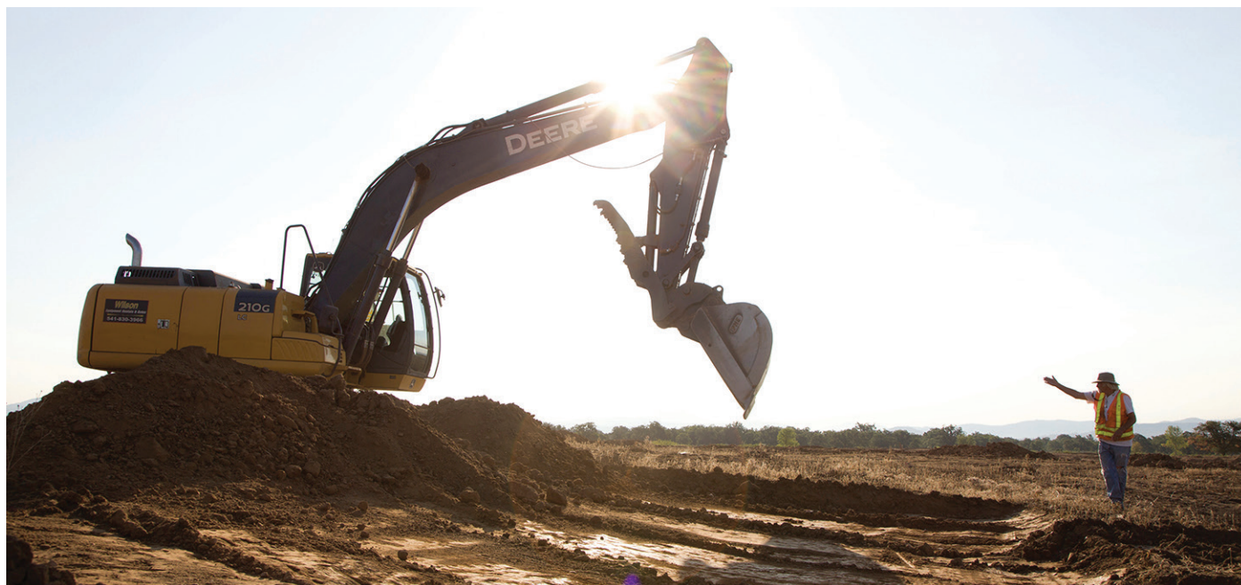
Working together, an equipment operator and ecologist remove upland soil from a filled vernal pool basin, using hand-signals and radio communication to adjust the depth and extent of excavation. © Evan Barrientos/TNC
