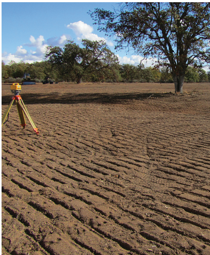
Track-walking imprints from a bulldozer's cleated treads line the restored terrain. The operator uses the weight of the machine to stabilize and settle the soil after final grading. © Keith Perchemides/TNC
