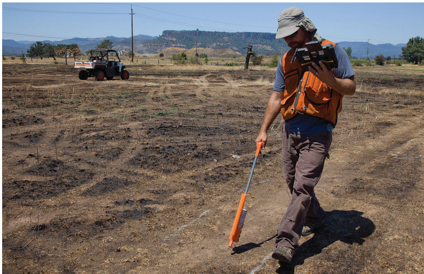
Marking out a vernal pool basin perimeter for excavation using construction marking paint, guided by the restoration grading plan on a survey-grade GNSS tablet. The area was burned earlier in the season to clear vegetation. © Evan Barrientos/TNC
