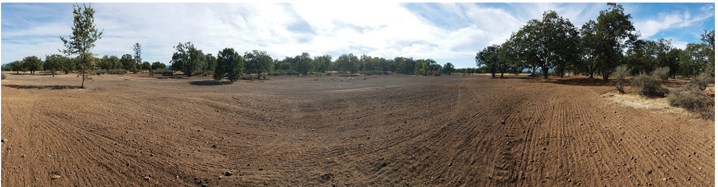
Newly restored terrain in late summer just after final grading. Track-walking followed by chain-harrowing stabilizes soils and provides an ideal fine-textured seedbed for fall sowing of native plant seed. © Keith Perchemlides/TNC
