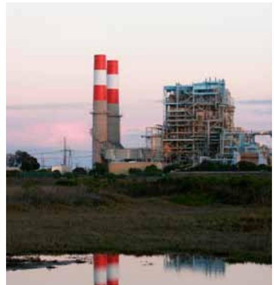
Vulnerable coastal infrastructure in Oxnard, CA
