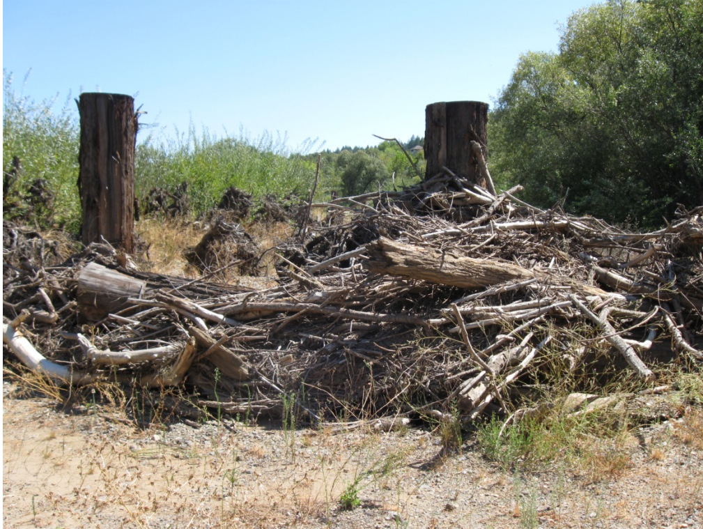
Photo 3. Woody debris that has collected in front of a constructed log jam at Reach 7.
