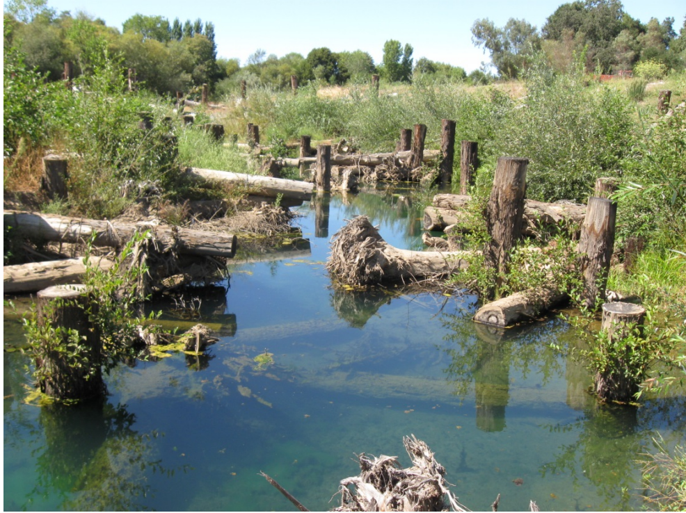
Photo 5. Close-up view of the backwater alcove constructed in 2013 as part of the Dry Creek Habitat Enhancement Demonstration Project Reach.
