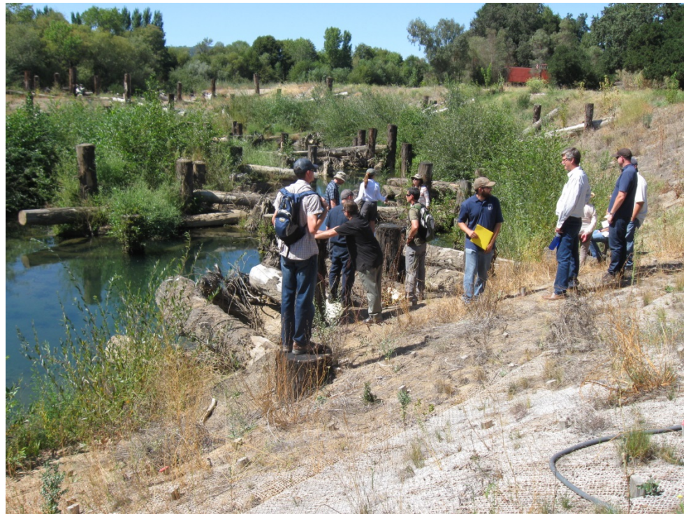
Photo 6. Wood for Salmon Working Group participants discussing the backwater alcove structure constructed as part of the Dry Creek Restoration Project.
