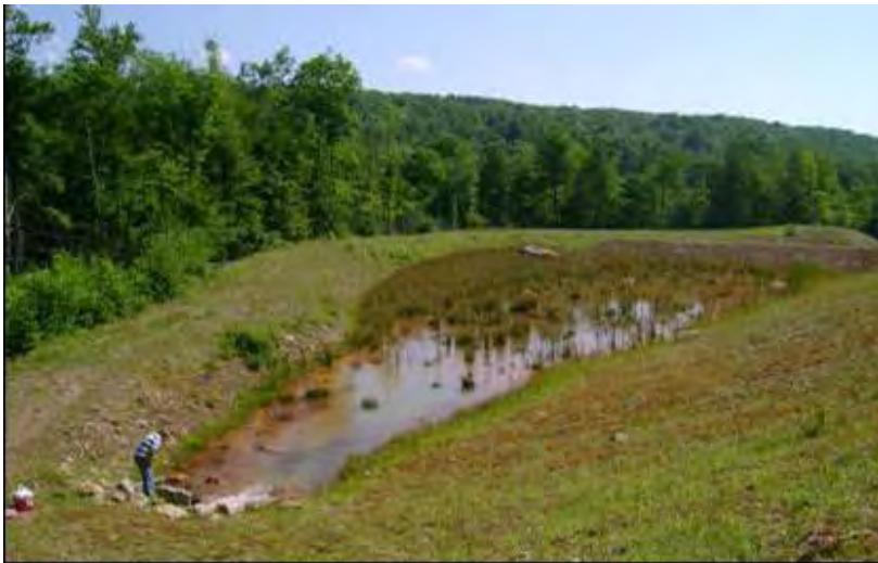
Passive Wetland Treatment System: Lausanne Tunnel water flows through pipes (forefront) into Wetland A (Photo: Wildlands Conservancy)
