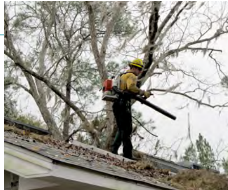
A forest ranger from the Florida Forest Service blows leaves from a roof as part of wildfire mitigation efforts. All photos: FFS
