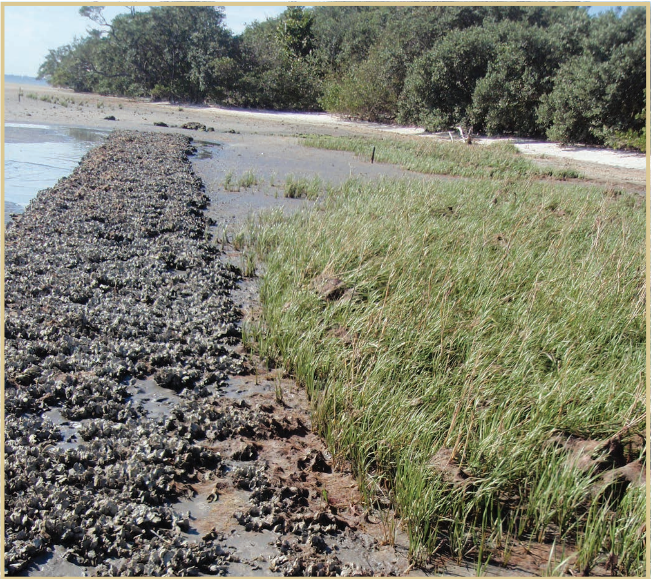
Figure 8: Oyster reef constructed to reverse erosion and promote sediment deposition and marsh growth, B. Hancock.
