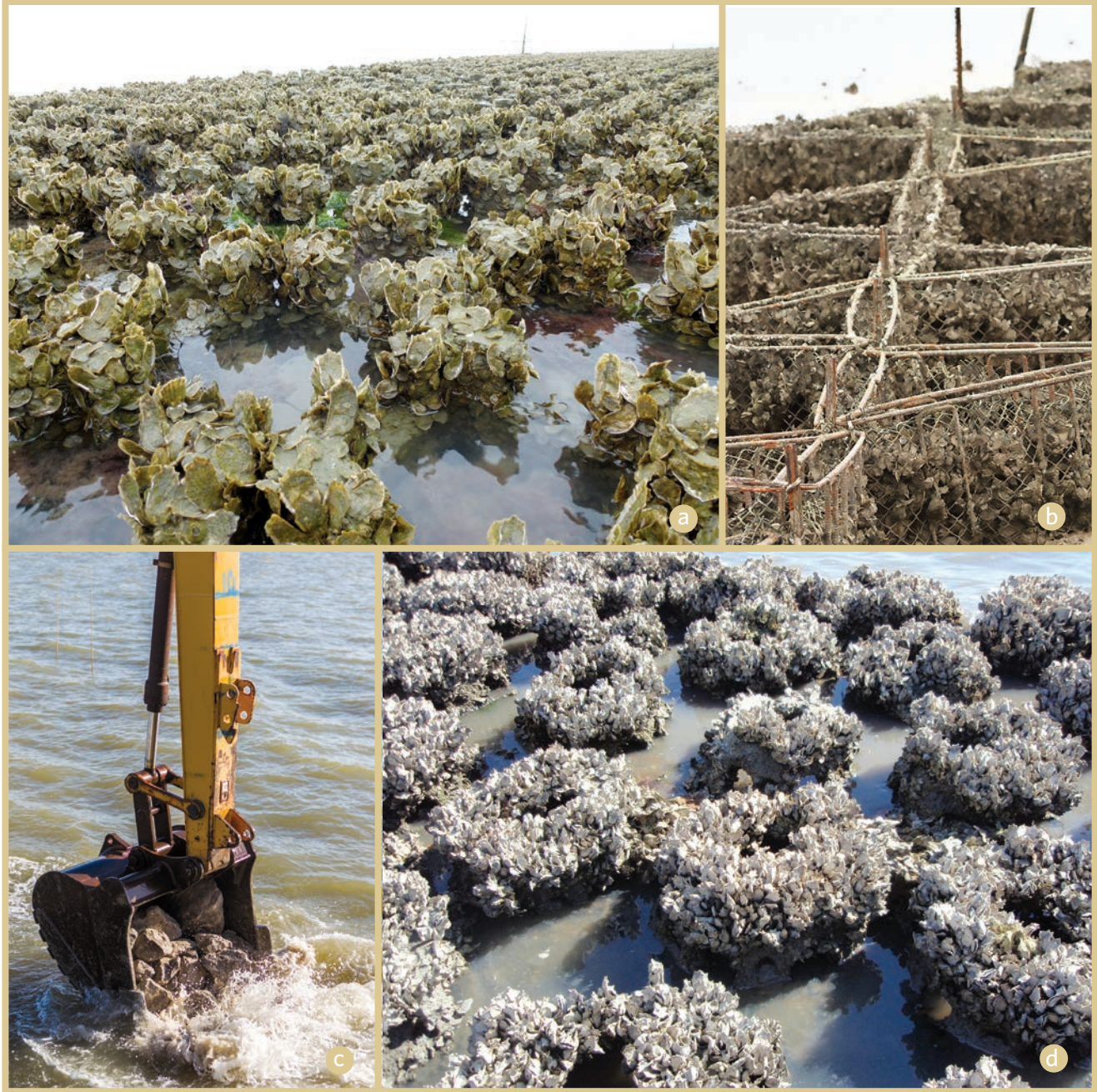
Figure 5: Artificial substrates used to construct oyster reefs, (a) cement castles VA, B. Hancock, (b) rebar frames TX, C. Smith, (c) limestone marl TX, J. Foster, (d) reef balls FL, B. Hancock.
