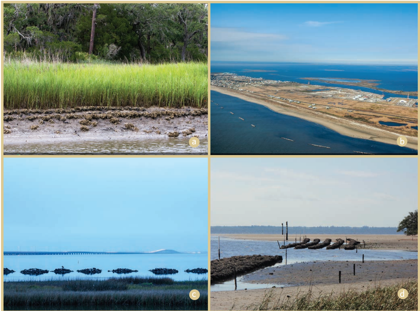
Figure 17: Some examples of oyster reefs constructed to assist in shoreline protection. (a, b, c) Erika Nortemann, (d) B. Hancock.
