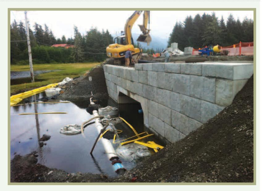
Construction of a larger culvert at the Klawock Highway. © Rob Bosworth, TNC
