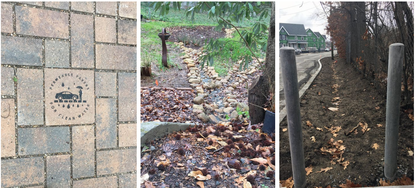
Examples of green infrastructure. (Left) Pervious pavement installation completed by the Mississippi Watershed Management Organization in Minneapolis, MN. (Middle) Rain garden facility completed by HABESHA in Atlanta, GA. (Right) Unplanted bioswale designed to accept and filter water from the adjacent roadway, part of Boston’s Slow Streets Initiative in Codman Square. All photos courtesy of David Queeley.
