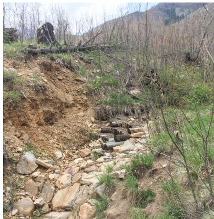
Local materials such as logs and rocks are being used for post-fire streambed erosion mitigation in the Manzano Mountains. © Forest Stewards Guild (Zander Evans)
