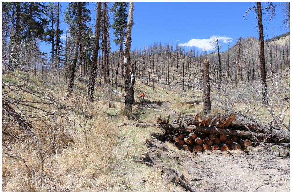
A sediment capture structure is constructed of burned trees.
